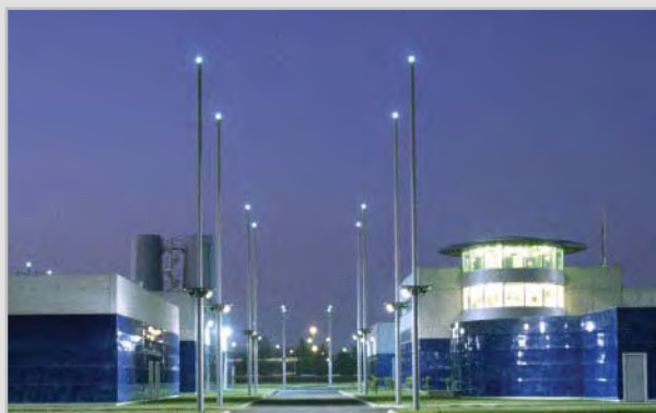
Station d'épuration Clos de Hilde © CUB
