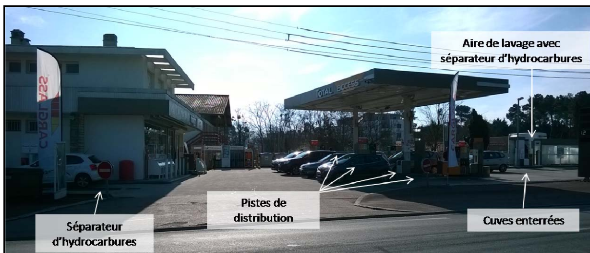
Figure 31 : Infrastructures pétrolières de la station service TOTAL ACCESS
