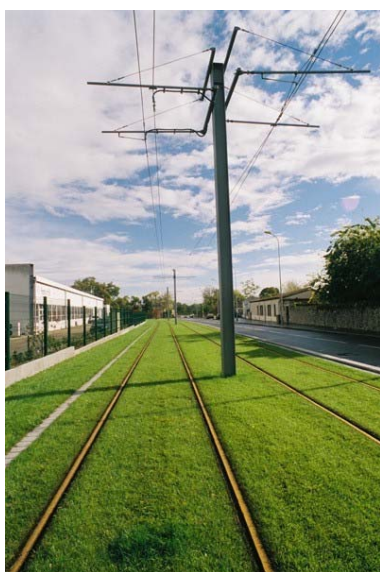
Ancrage Poteau axial
